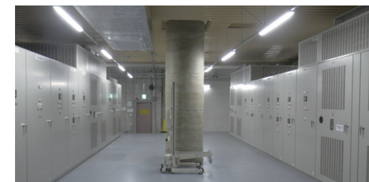
High/ low voltage switchboard (Ueno Station)
