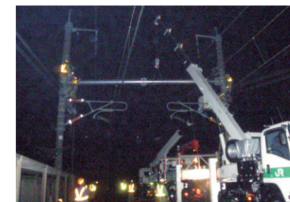
Aseismic reinforcement construction (new construction of beams)
