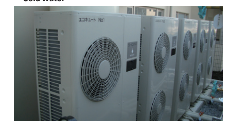
Heat pump water heater
