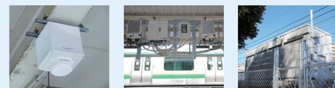
Antenna, Relay terminal device (slave station), Optical transmission device (master station)
