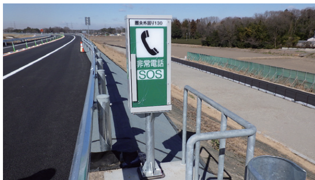
Installation of expressway emergency call box
