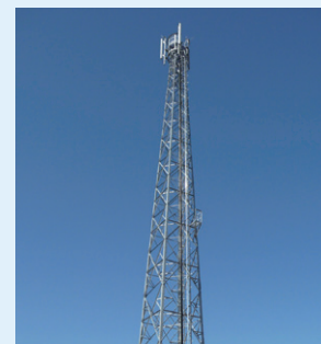
Mobile phone base station (steel tower)
